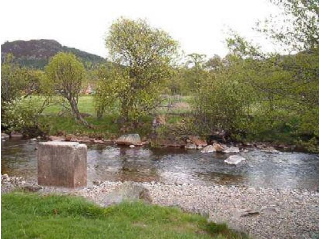
Fig 2 site for footbridge showing old pier from original bridge
